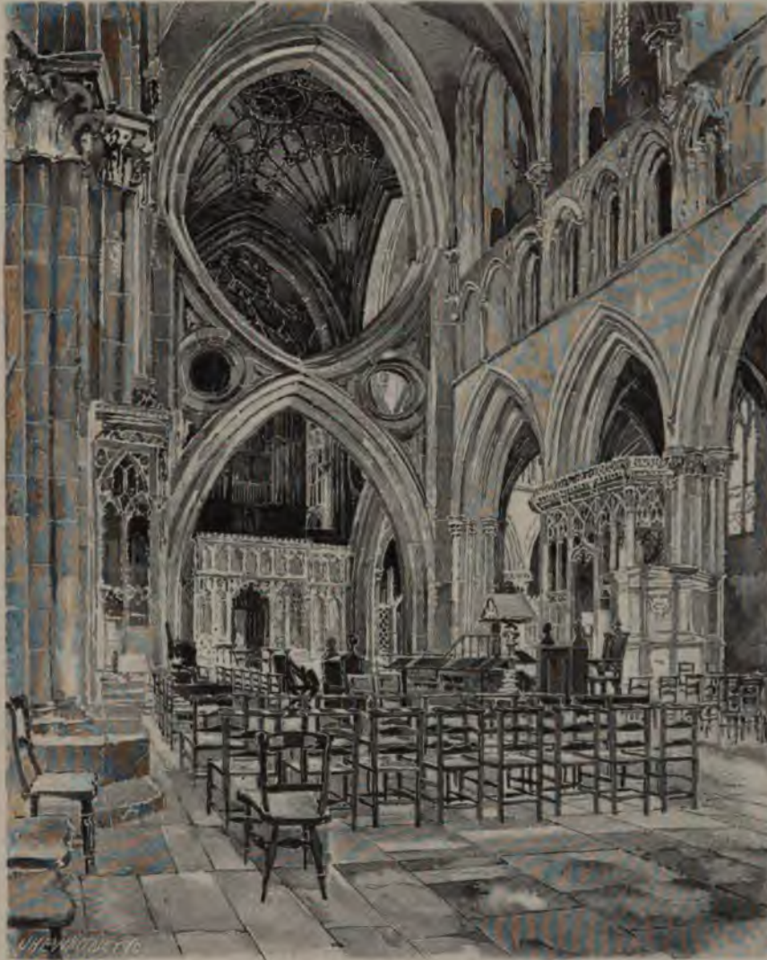
THE NAVE, LOOKING EAST.
